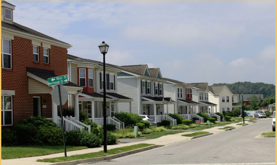
Gateway Crossing (HHA)
